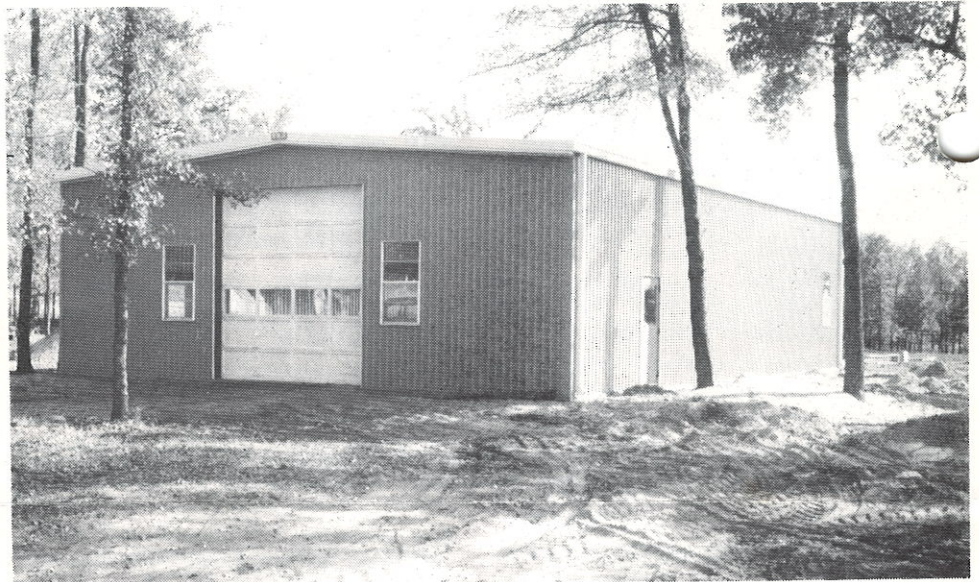
Spacious new garage constructed.
